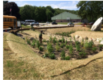
Bioretention basin installed near Giorgetti Park in the City of Rutland
