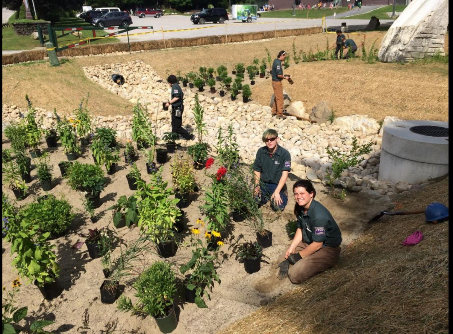
ERP funded VYCC crew plants the bio-infiltration basin
